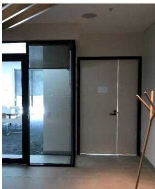
Photo 5.4 – Access door in ADG offices
