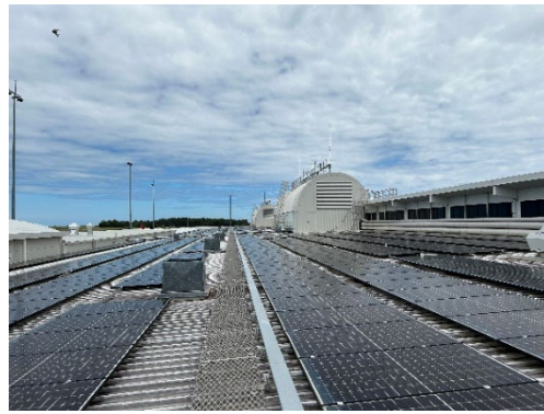
Photo 6.3 – Area A – looking west
