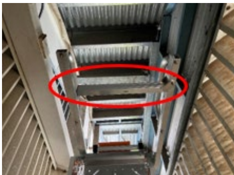
Photo 6.31 – Area Central PR filter – Guard rail closed
