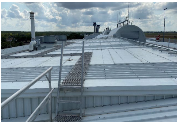
Photo 6.20 – Area D – Step access Area B to Area D West
