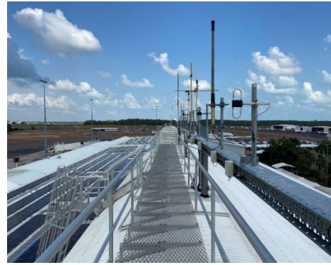
Photo 6.28 – Area PR – Radiation Hazards
