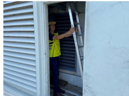
Photo 6.30 – Area Central PR filter – Correct ladder discipline
