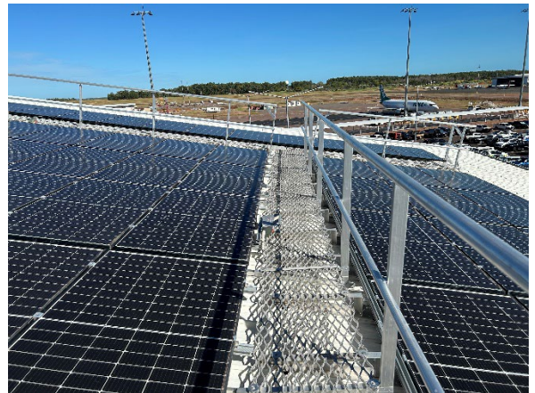
Photo 6.9 – Area B West – Roof walkways looking West.
