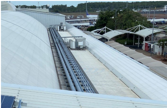
Photo 6.17 – Area C – Viewed from Area B East
