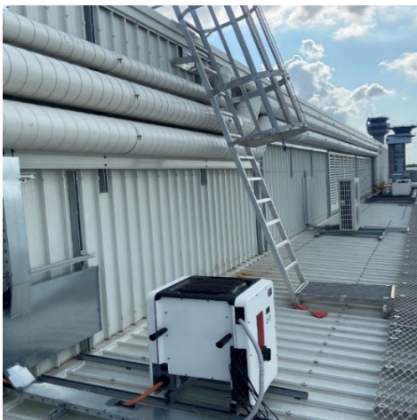
Photo 6.14 – Area B East – Locked Ladder - Area A to Area B East
