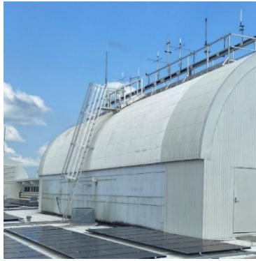
Photo 6.27 – Area PR – Ladder view from Area A to PR
