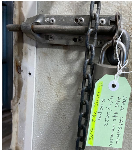
Photo 1 – Terminal roof access door is locked in the open position when you access the roof
